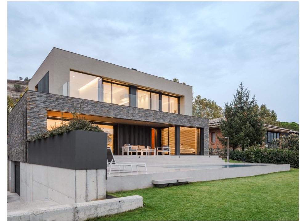
PROJECT: SANDRA SOLER STUDIO / PHOTO: MARC TORRA
